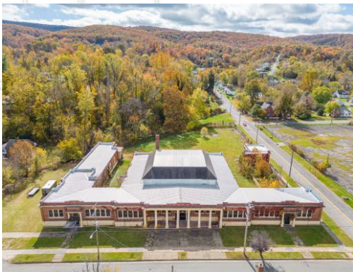
Pilot project is Pulaski, VA: Historic Jefferson School to be restored and adapted for vertical farming
